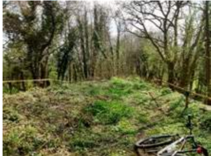
Path to be constructed in the centre of Bridge 11. Install new railings, Standard route 2.5m wide with horse construction
