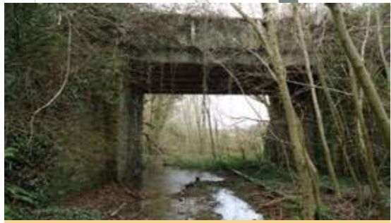
Bridge 12. Access ramp to be formed to link with Bridleway
