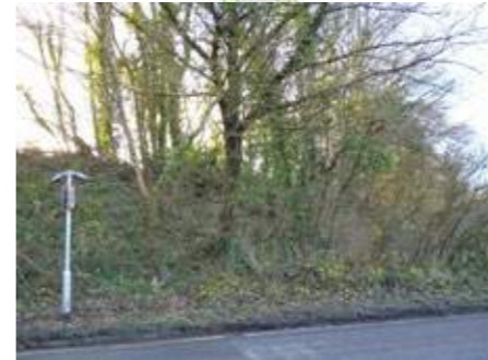
Ramp constructed into the existing railway embankment. Gradient 1:20 so approximately 70m in length wide enough for 2.5m wide path and horses in verge
