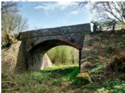
Bridge 10. Ramp from road down to railway formation
