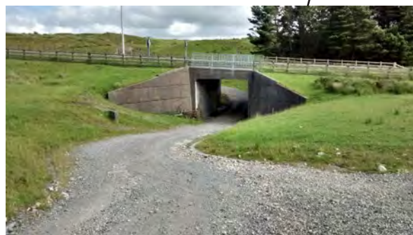
Route passes through existing underpass underneath A465 slip road
