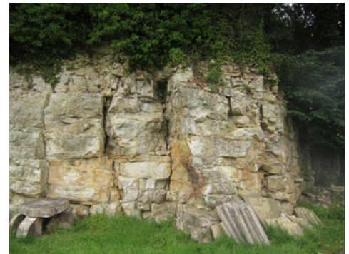
An exposed rock face
