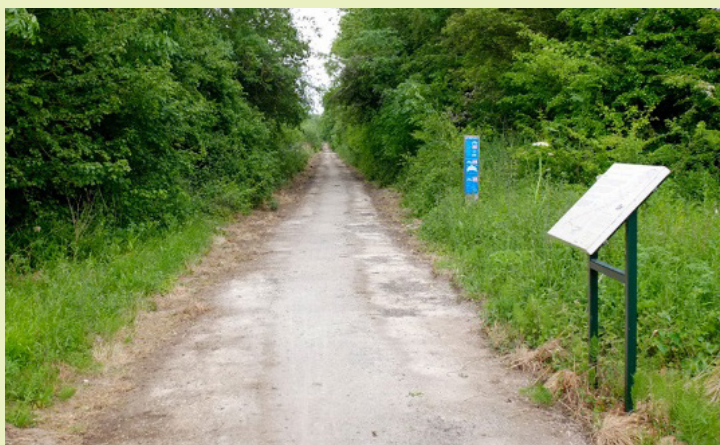
Path after 'scraping back' edges
