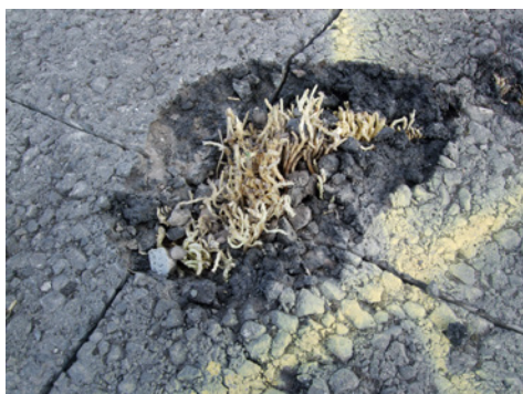
Do not pull weeds growing through the path surface, use herbicides if necessary
