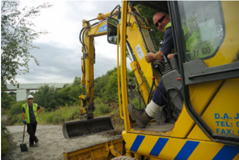
Route construction underway
