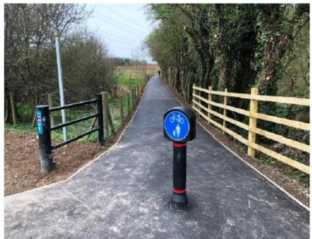
Photo 2: Restrictive chicane replaced by a single bollard on National Route 15 in Grantham, Lincolnshire © Sustrans 2019
